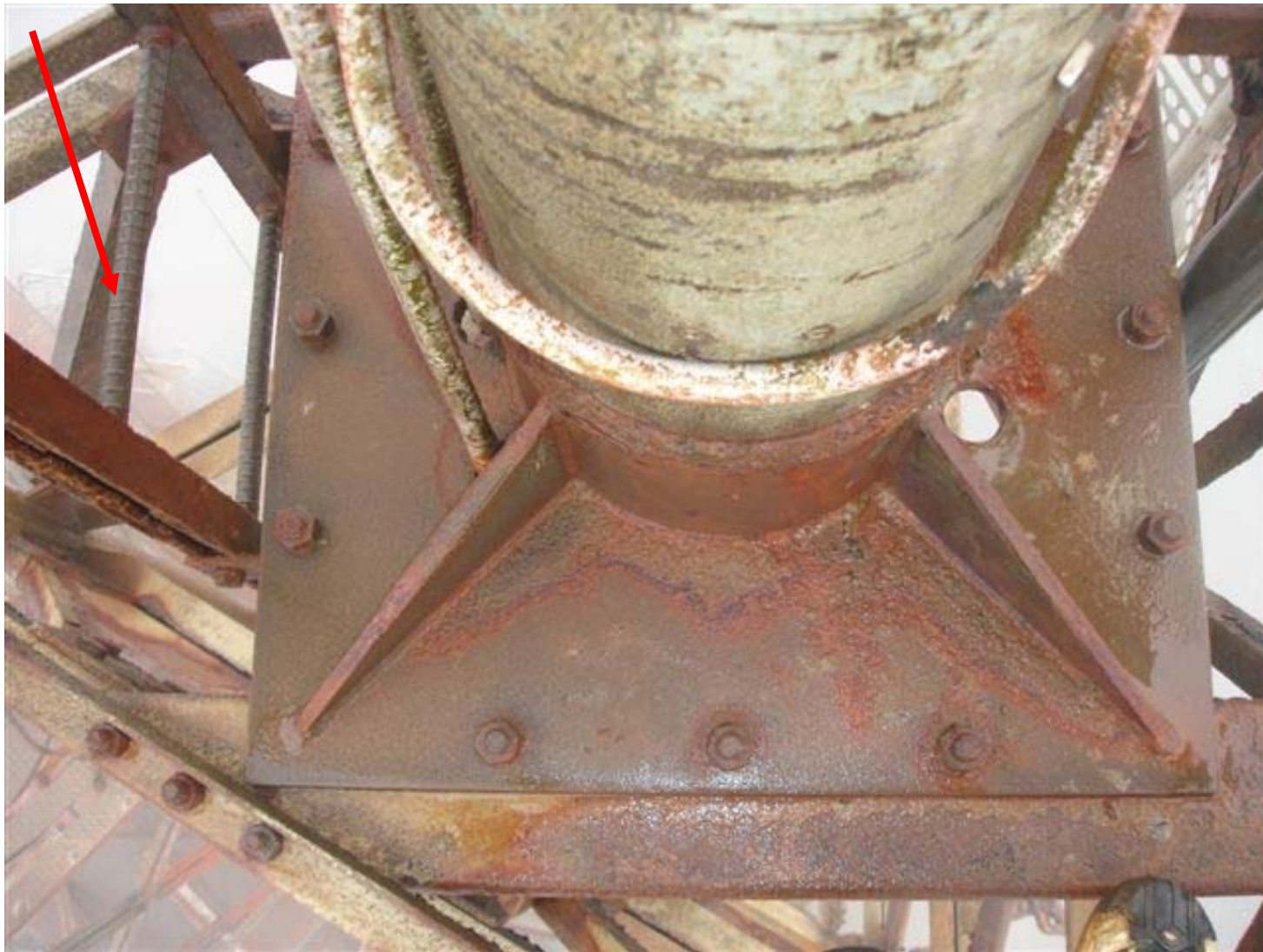
Top section of tower and bottom bury cup. Note new rebar ladder.
